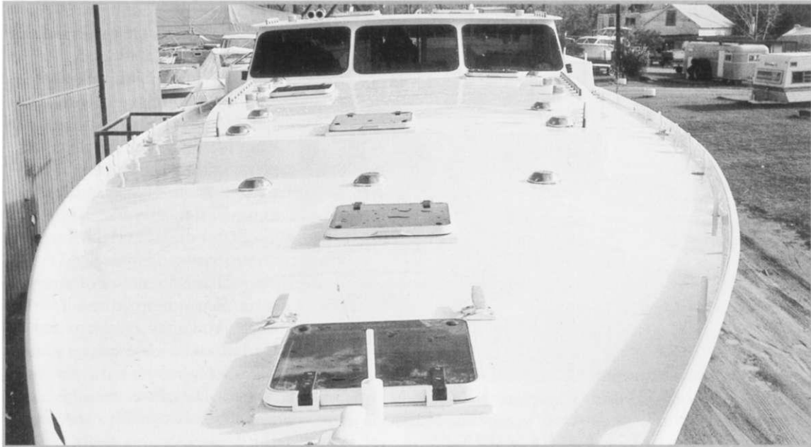
The steel deck on this Roberts 64 is now ready to receive a laid wooden deck or one of many other alternative treatments.
