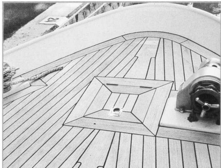
This 1-inch (25 mm) teak deck has been in place for 15 years; some recaulking has probably been necessary. Note the low bulwark, ably supported by a pipe caprail.
